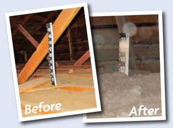
Varna's attic had less than an inch of insulation prior to the Energy Efficiency Makeover. Matt Hoisington, C&V Home Improvement, increased the insulation to the recommended 10-12 inches.
